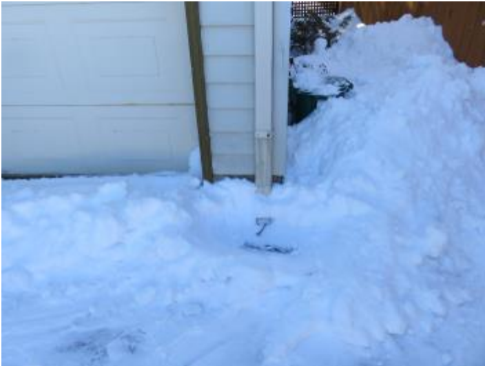
Figure 9 NW Downspout Discharging onto Walkway(s) Figure 10 SW Downspout Missing Extension
