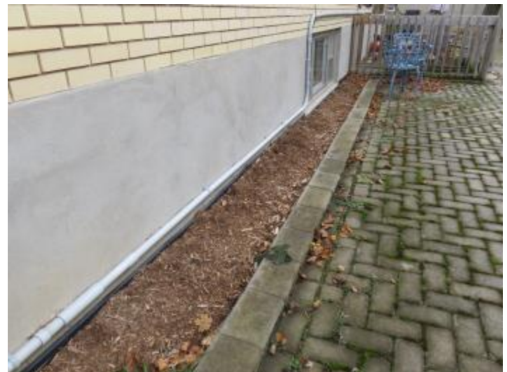
Figure 6 Exterior Waterproofing at Back of Building
