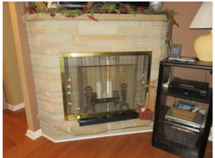
Figure 16 Recommend Specialist Evaluate Fireplace
