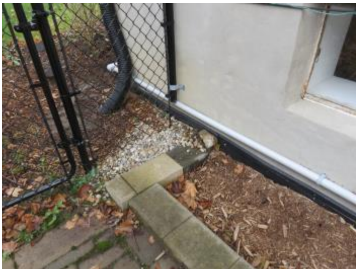
Figure 5 Exterior Waterproofing at Back of Building
