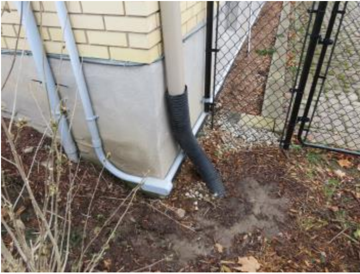
Figure 9 NE Downspout Discharges Below Grade
